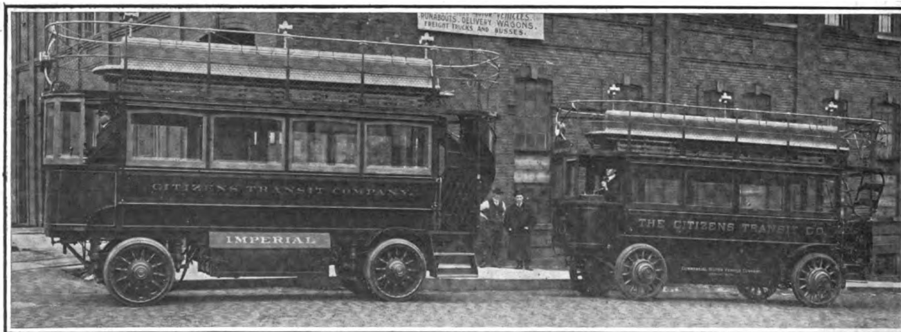
DOUBLE-DECK ELECTRIC OMNIBUSSES CONSTRUCTED BY THE COMMERCIAL VEHICLE COMPANY IN DETROIT
